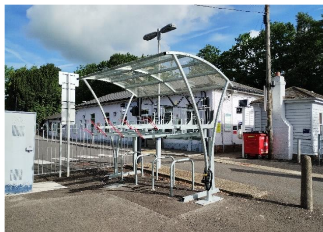
The new position of the cycle rack at Hildenborough station
