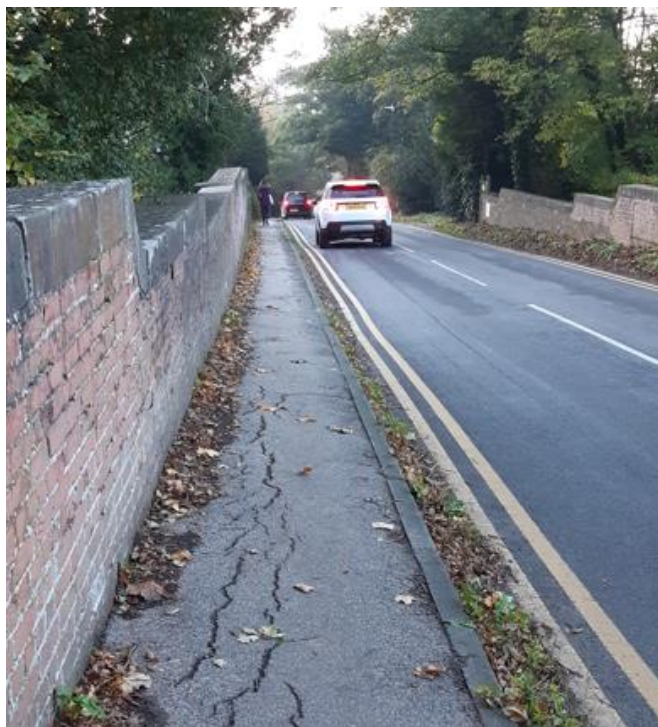
The pavement is narrow on the bridge out of the station
